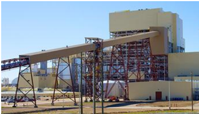
The 600-MW John W. Turk, Jr., Power Plant in southwestern Arkansas exemplifies our commitment to the responsible use of coal as a fuel source.
