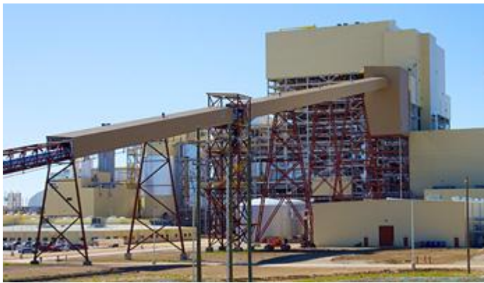
The 600-MW John W. Turk, Jr., Power Plant in southwestern Arkansas exemplifies our commitment to the responsible use of coal as a fuel source.
