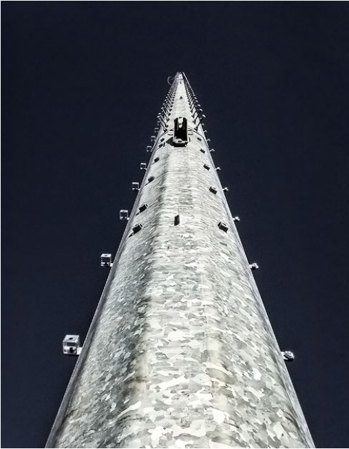
Looking up at the 120-foot pole at Elcona Station in Elkhart, Ind. The station is part of Indiana Michigan Power's volt var optimization project, a distribution automation system.
