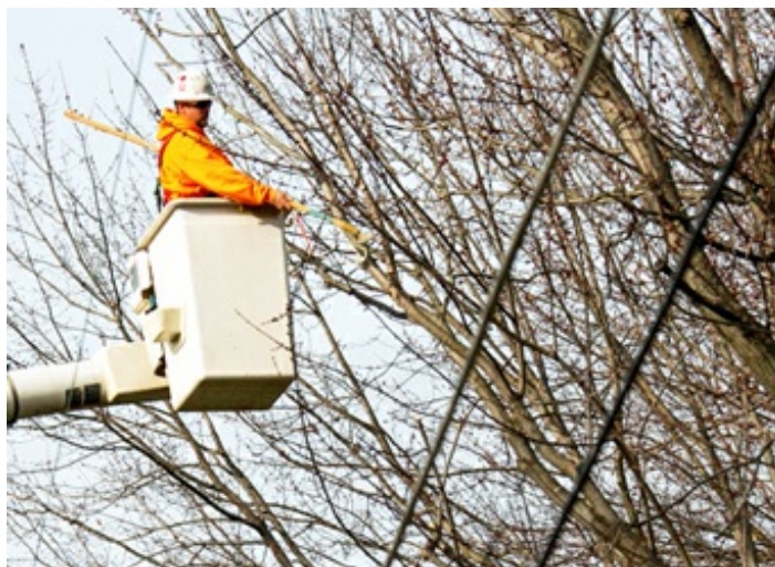
Managing vegetation on our rights-of-way is a key to maintaining transmission and distribution system reliability.
