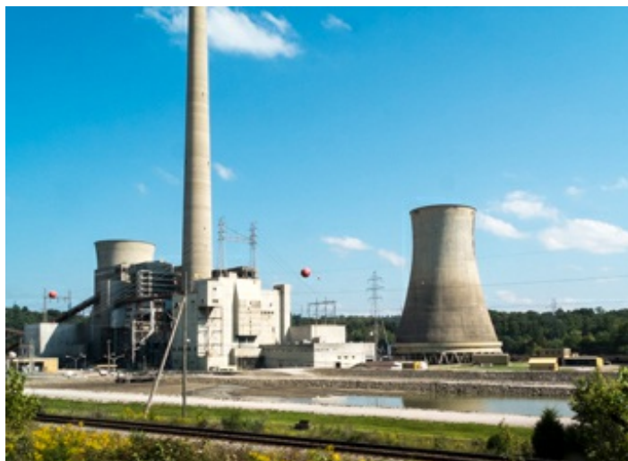
In June 2016, Kentucky Power Company's Big Sandy Plant completed its conversion from a coal-fueled generating facility to natural gas.
