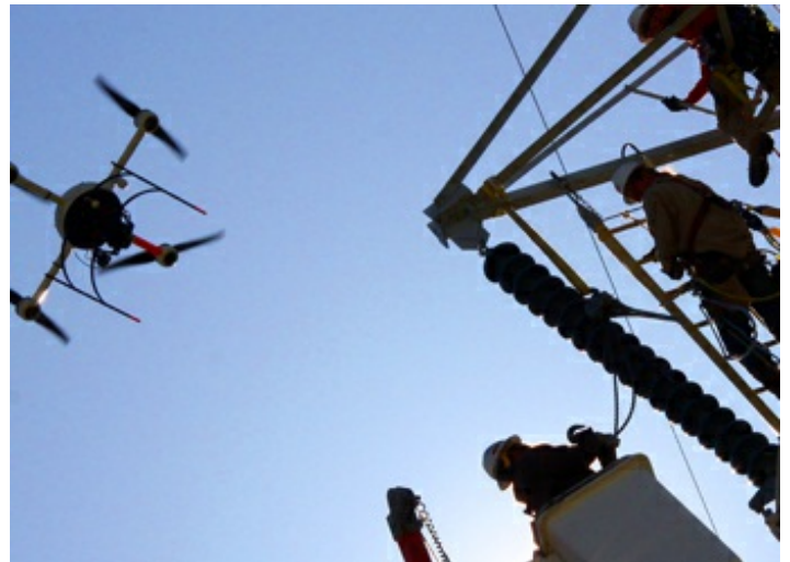
The use of drone technology is beneficial for a variety of inspection applications across our generation, transmission and distribution system.
