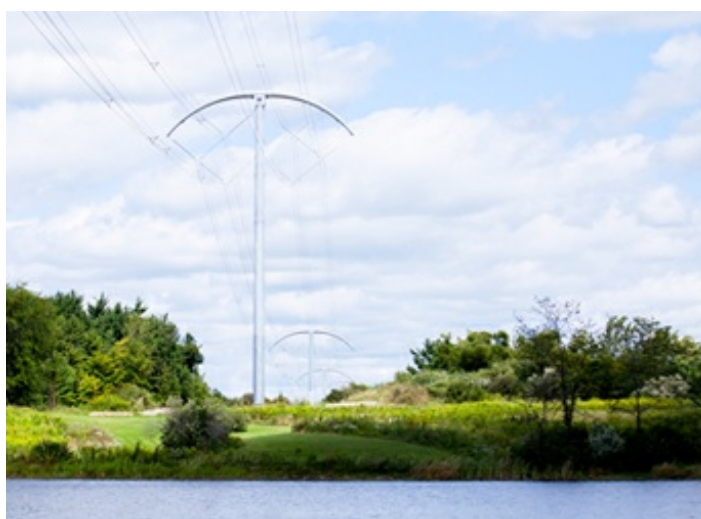
The compact BOLD 345-kV design provides advantages such as lower tower heights and increased capacity in the same right-of-way.
