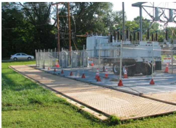
AEP uses prefabricated packages to build transmission substations more
