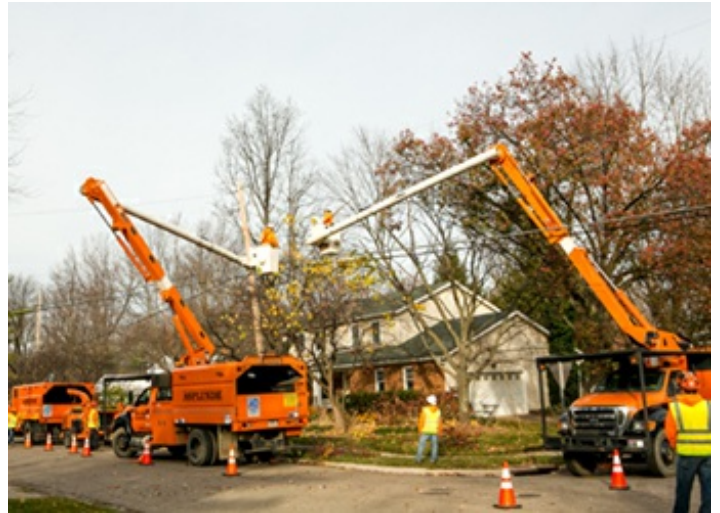
Vegetation growing into and trees falling onto power lines are the major cause of power outages which is why managing vegetation in and along our rights-of-way (ROW) is part of our strategy for maintaining system reliability.
